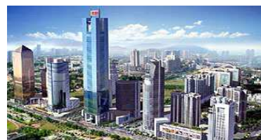
Guangzhou, Lines 4 and 5
